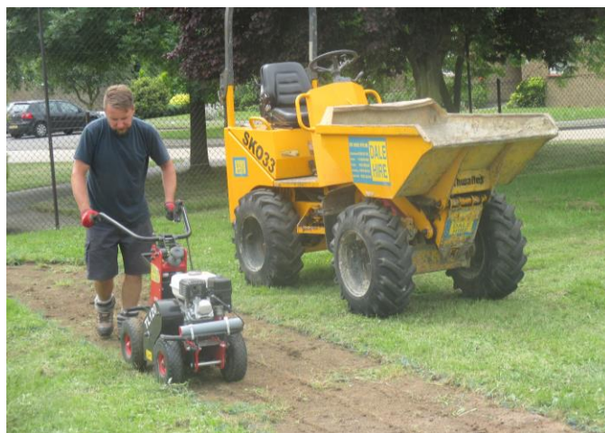
Digging out the foundations for the track
