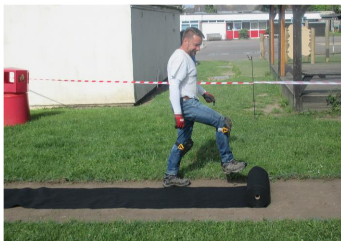
Laying the membrane matting so that weeds and grass do not grow through the track.
