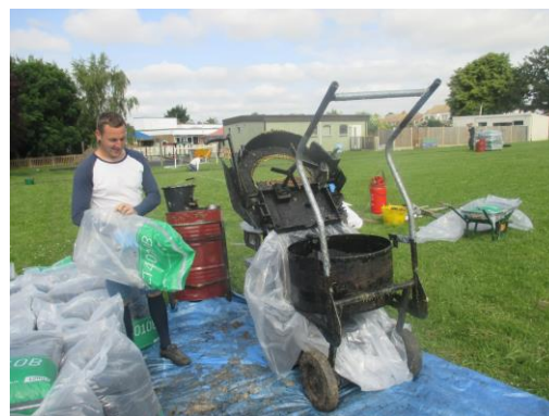
Mixing the rubber material ready to lay. The material is made from recycled car tyres.
